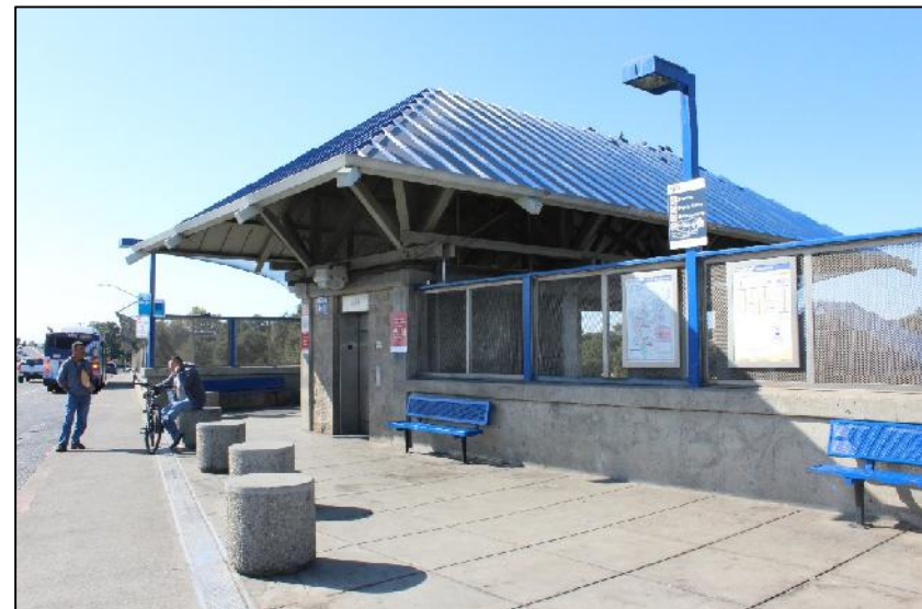
Southbound bus stop on Watt Avenue.
