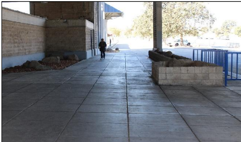
Riders transferring between the northbound bus stop and light rail feel unsafe walking under the overpass area.
