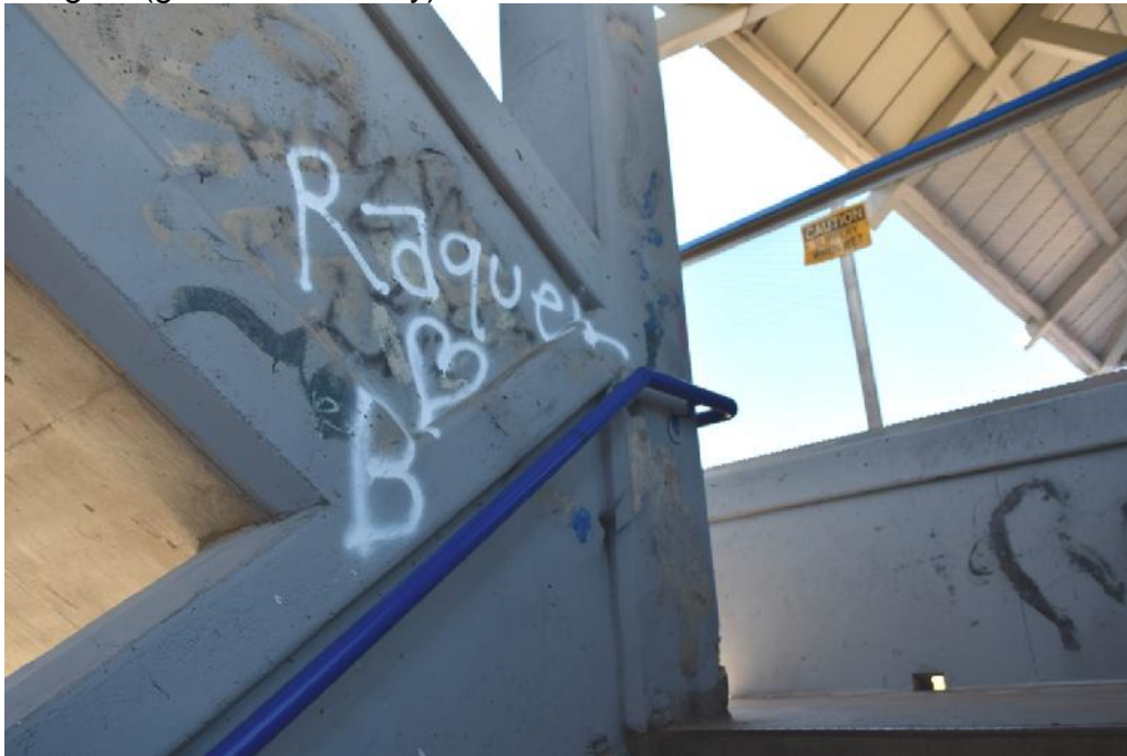
Image 9 (graffiti in stairway)
