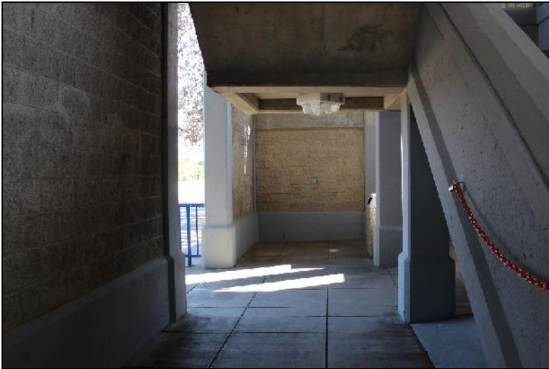
Redesigning the staircases and elevator shafts can reduce hiding spaces to improve natural surveillance.
