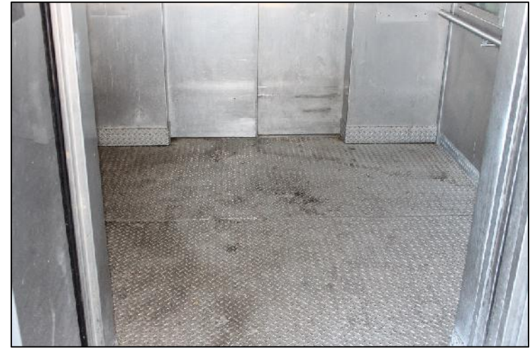
Unsanitary elevator conditions contribute to an unpleasant transferring experience.
